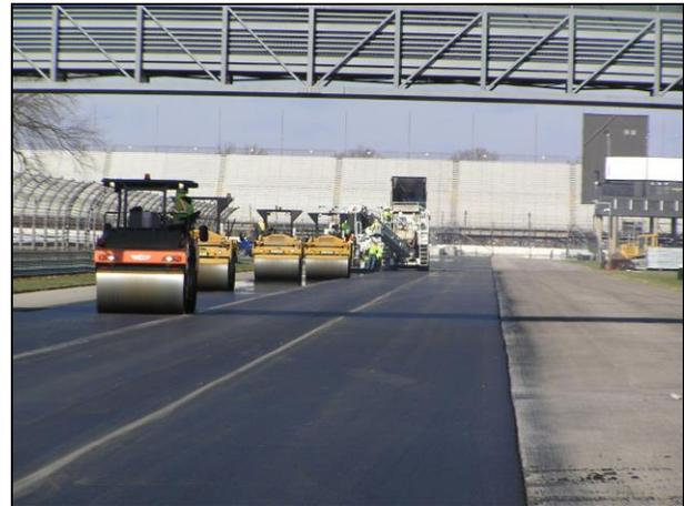
*Placement of the 9.5 mm steel slag surface course on the road course in the center of the IMS infield, looking north, parallel to Hulman Boulevard.*
