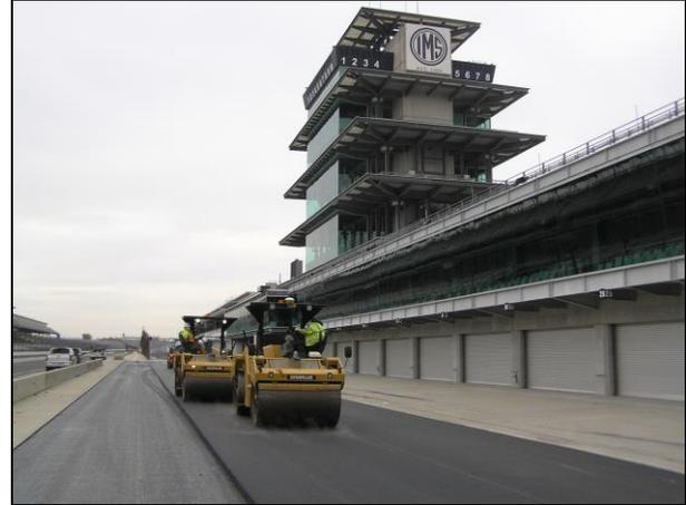
*Placement of the 9.5 mm steel slag surface course in front of the IMS Pagoda and MotoGP Garages.*
