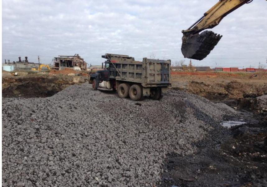
The uses of steel slag are diverse, as it can be used for general backfill, ground improvement, road base, foundation and slab support, etc. It can also be processed into various gradations and screened for particular applications. SESI specifies its use for venting layers in landfill gas systems and other similar depressurization systems.
